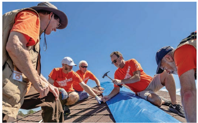
Tarpping damaged roofs helps protect homes for the weeks or months it takes to repair and make homes livable again.
