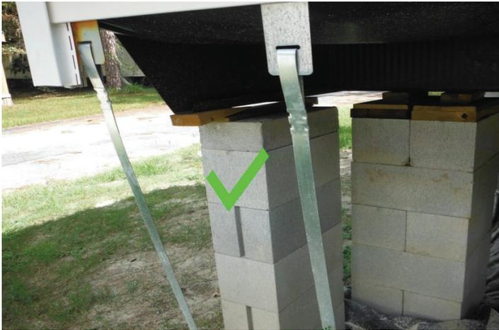
The second tie-down type of anchoring that may be added is attached to a home's vertical tie connector, or overhead strap. Many homes are manufactured with these connection points built within the siding of the home. Where possible, installers will add straps to these points as well.
